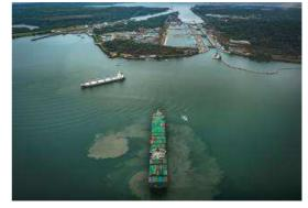
capacity of the largest size vessels that can cross the old locks. The new locks accommodate neopanamax ships that can carry up to 14,000 containers. A ship with this capacity pays approximately US\$850,000.00 in toll fees to cross the Panama Canal. The new locks were designed to reuse up to 60% of the fresh water that would flow into the ocean by using recycling water basins.
